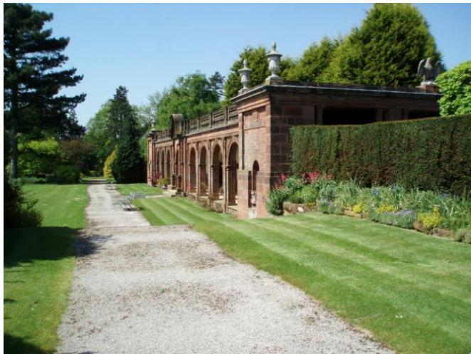
The loggia at Thornton Manor with principal red sandstone facade facing south west beside one of the main walks in the garden Photograph Barbara Moth
