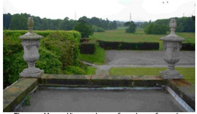
Thornton Manor: View south west from the roof over the garden and parkland towards the Dee estuary and north Wales Photograph courtesy of Maria Luczak
